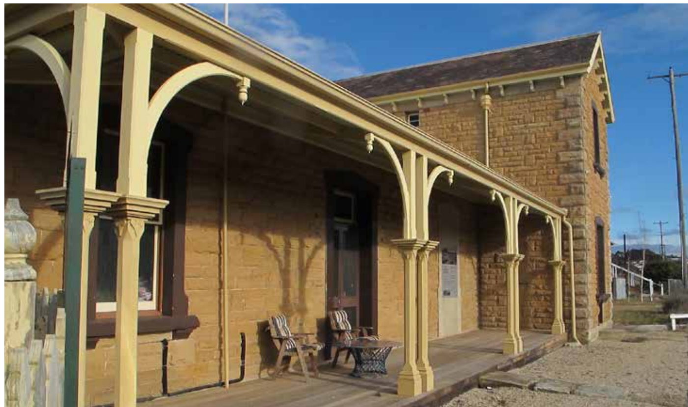
View of the north east side of the Wallerawang railway station (c.1870) façade. (Gina Scheer, 08.06.2016)
