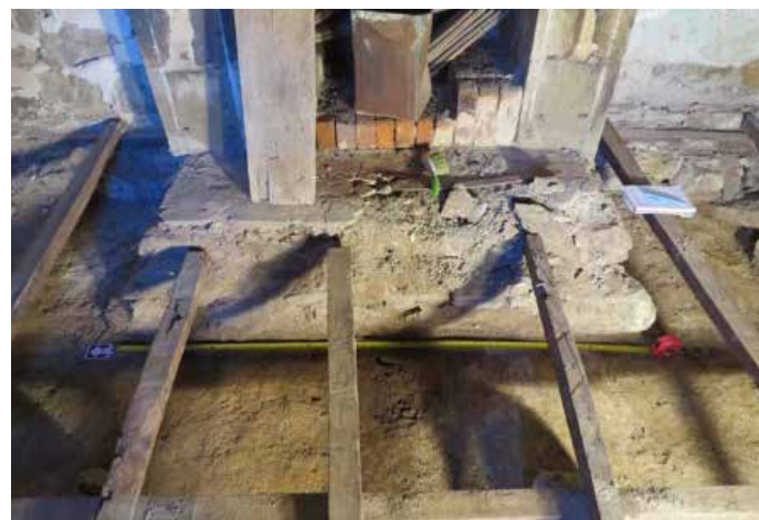
Room 3 fireplace area after underfloor archaeological excavation. The stone bearers and timber joists were retained to help identify room areas for later artefact analysis.
