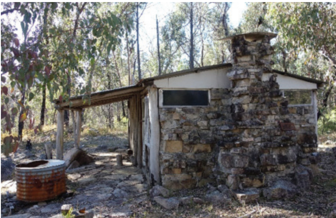
Another view of Franks Hut, eastern wall with granite stone fireplace
