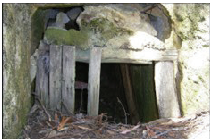
Figure 3: 2004 photograph of entrance to tunnel showing wooden frame and slats.
